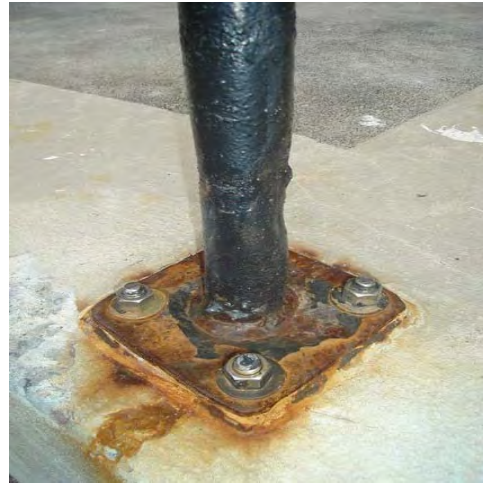
Corroded post
