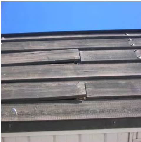
Warped wood siding
