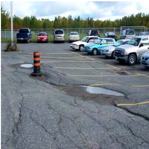
Original 30 year old roadway
