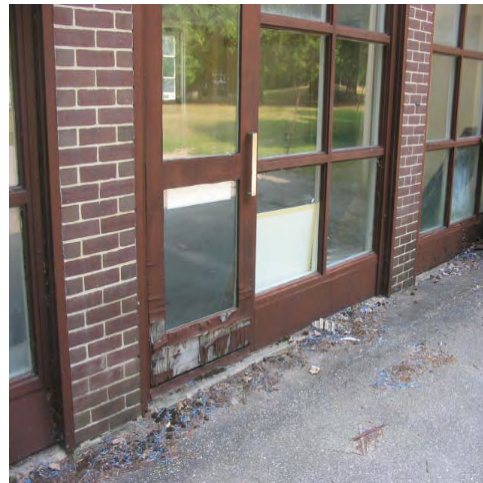
Moisture Damage
