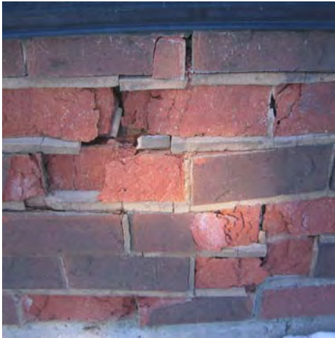
Spalling Brick
