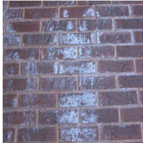
Efflorescence
